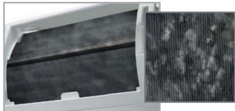
The main cause of odour within air conditioners is mould and bacteria in the heat exchanger. When the indoor coil is wet, organisms breed, creating odours.
